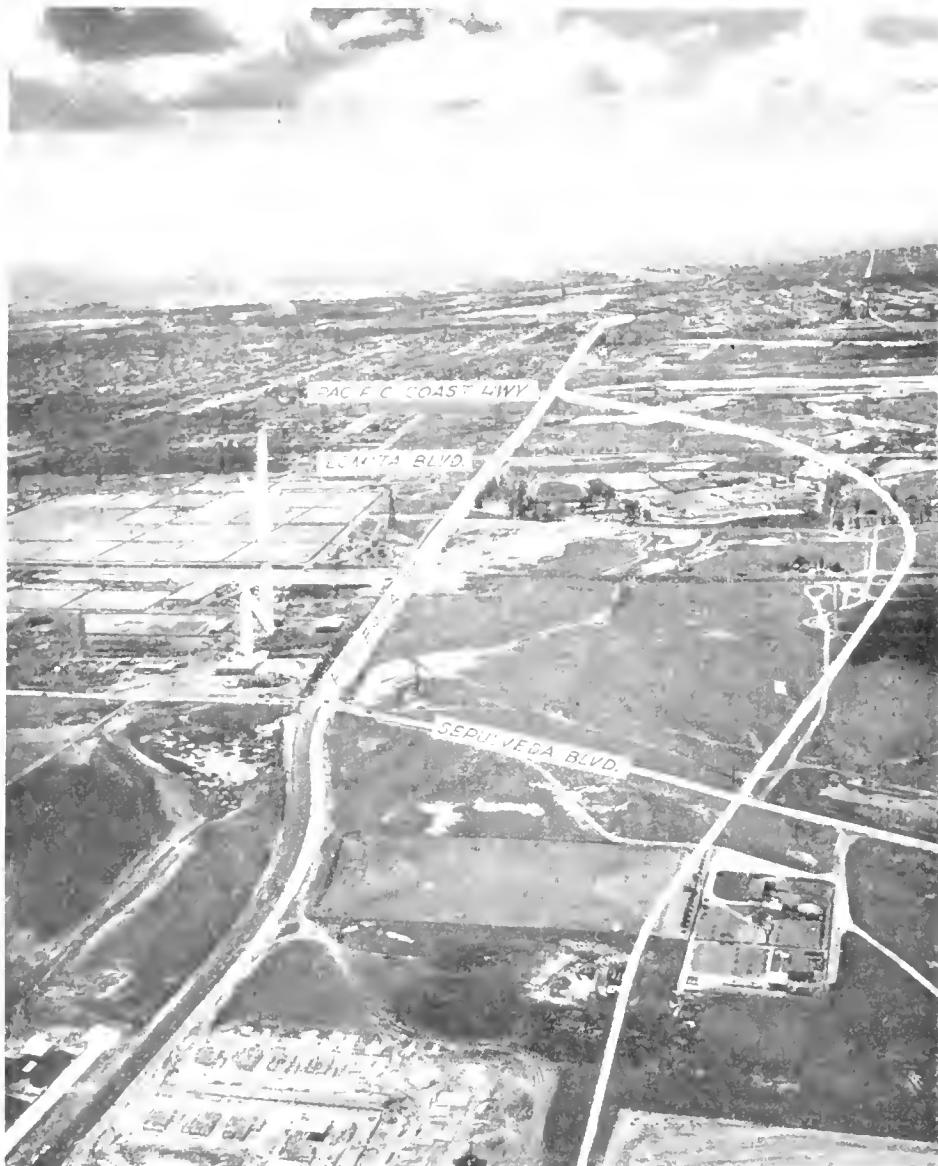
Looking southerly along routing of Harbor Freeway with Los Angeles Harbor and Pacific Ocean in background. Los Angeles County Sanitation Plant appears center right inside loop of freeway location.
